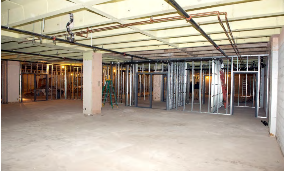
Figure 3. Construction as the walls begin to define the space
