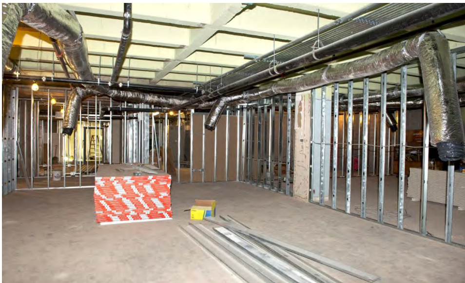
Figure 4. Construction as the HVAC goes in
