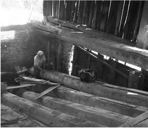
Figure 9.—Floor joists from a hay press barn located in Braytown, Indiana (Switzerland County). Note the author straddling a floor joist that is constructed from an entire tree bole.
