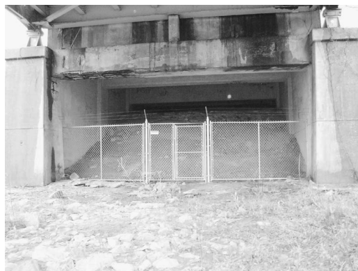
Figure 3.—Photo of north side of bridge.
