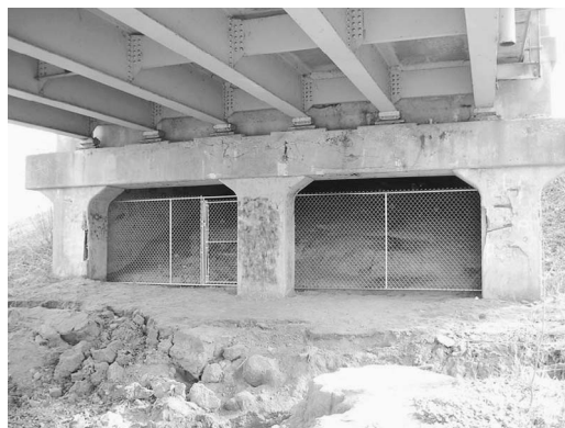
Figure 4.—Photo of south side of bridge.
