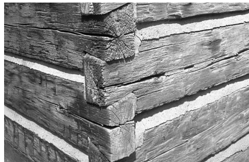
Figure 4.—Close up of southeast corner of the Grayson house showing half-dovetail notching.
