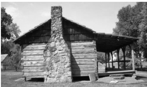
Figure 3.—Grayson house east façade showing end chimney and porch.
